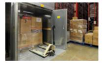
Ensuring safe and easy stock-movement is key to running a business efficiently. Available as goods-only lifts or goods lifts with an attendant, these lifts offer the perfect, cost-effective solution for transporting goods between floors with a selfsupporting structure and minimal pit.
