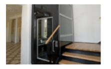
Our passenger platform lifts offer similar solutions to our vertical platform lifts, suitable for low rise buildings, travelling up to 9 metres. With two-panel side opening doors, these lifts are hydraulic rather than incorporating screw-driven drive technology and are available in a range of finishes and colour schemes.
